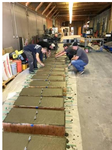
Checking rebar positions and eye bolt placement.
