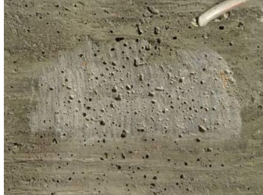
Gage area after grinding with many small voids.
