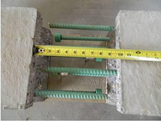
10 in. between precast interfaces.
