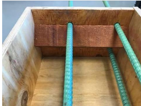
Shear key formwork coated with concrete surface retarder.
