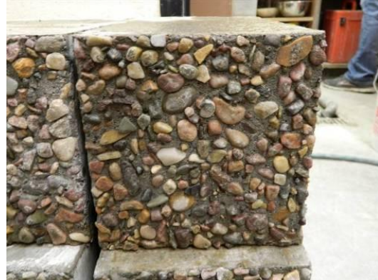
Exposed aggregate surface finish on the precast concrete.
