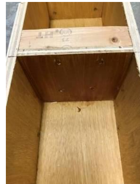
Concrete surface retarder applied to center divider.
