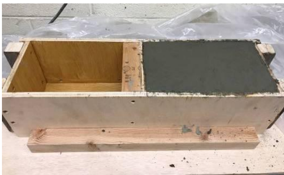
Precast concrete section poured.
