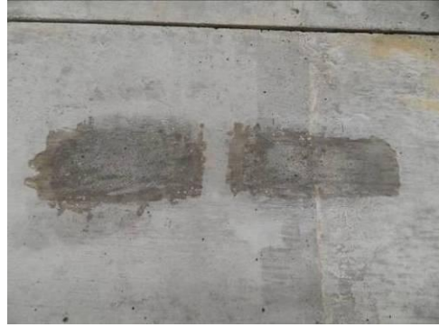
Grinding/sanding base coat down to concrete surface.
