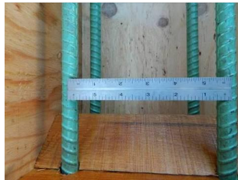
Showing rebar spaced 6 inches on center.
