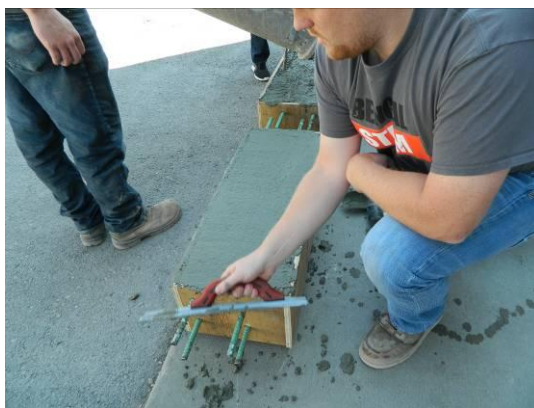
Finishing the surface with a trowel.
