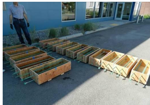
LB molds prepared for pouring.
