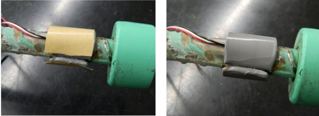
Figure L.12 Applying Rubber
