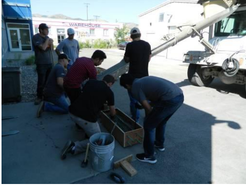
(a) Pouring large beams
