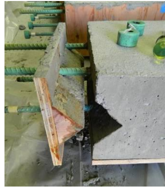
Removing shear key formwork.
