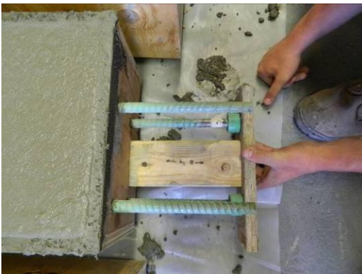
Checking the position of the rebars with wood gauge.
