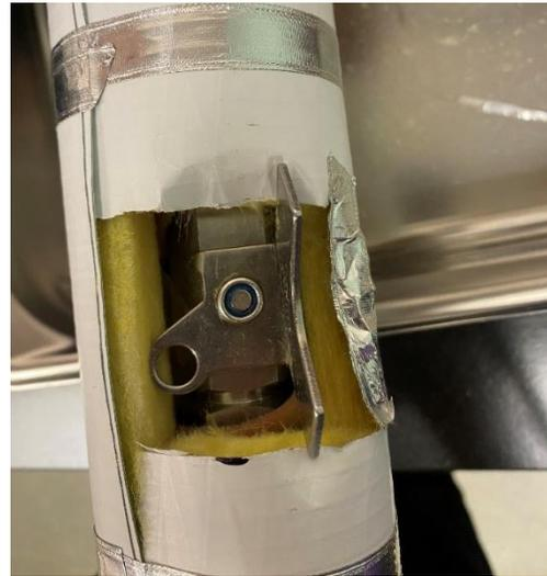
d) Ball valve handle is seen protruding through fully installed 12.7 mm ( $\frac{1}{2}$  in.) insulation.
