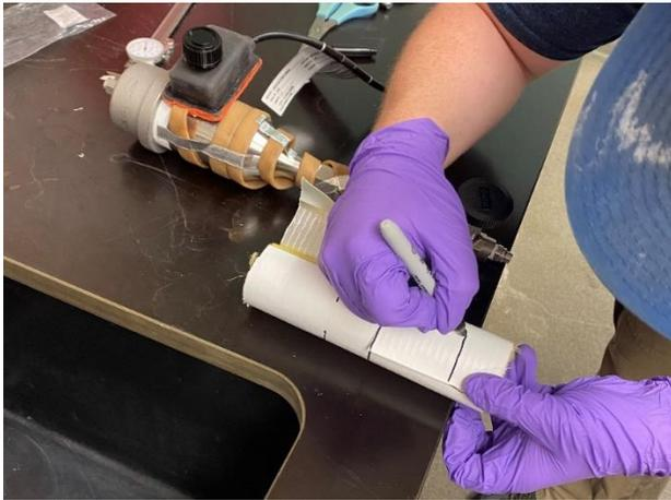
a) The insulation was measured and marked for the valve handle and stem cutout locations.
