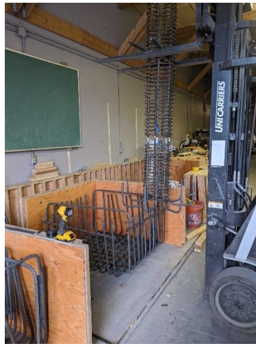
b) Placing of Pier Cage
