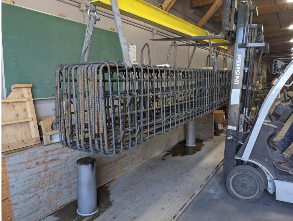
Figure 4-12: Cap Rebar Cage Placement
