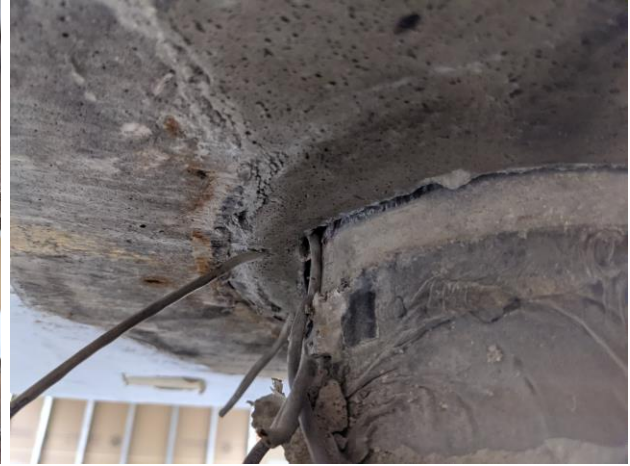
b) HSS and Grout Separation
