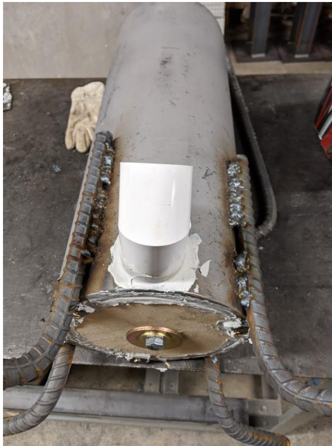
Figure 4-9: Embedded HSS Pipe Prepared for Install
