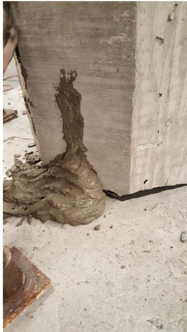
e) Grout flowing out of grout vent
