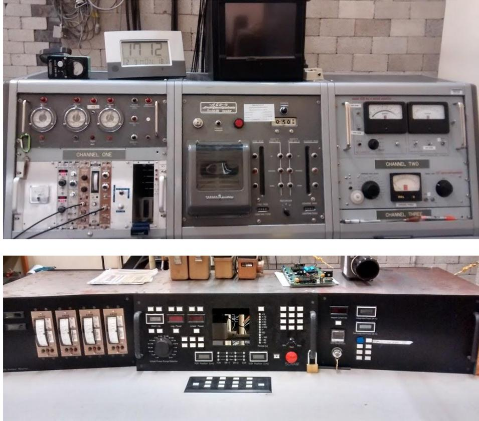
Figure 1. ANG-201 Control Consoles: Original (top), New (bottom)
