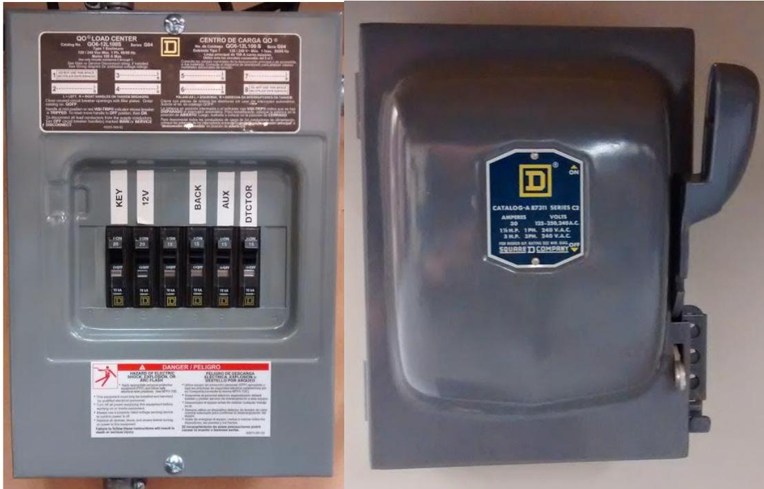
Figure 6. Breaker Box (right) and Kill Switch (left)
