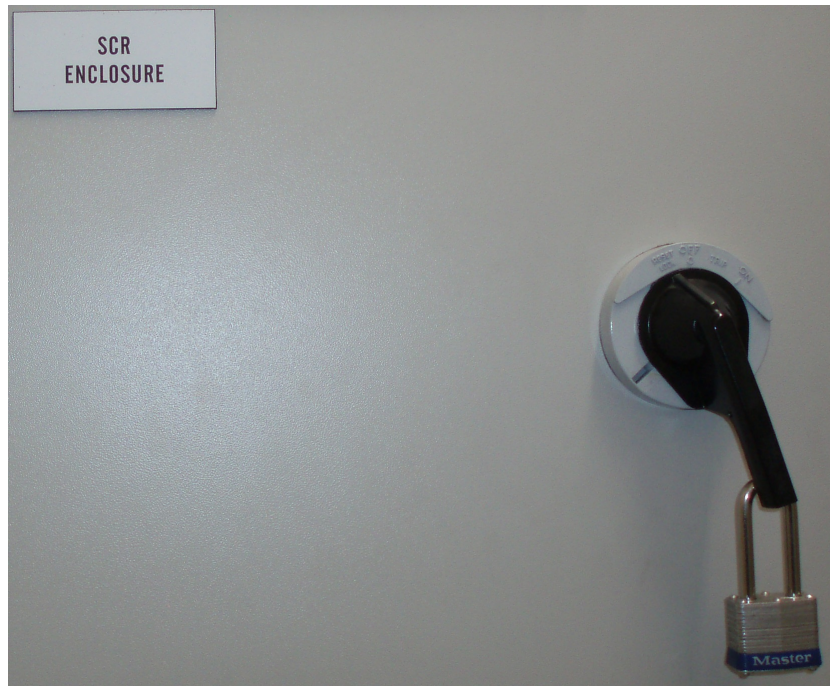
Figure C.2: SCR enclosure and the padlock.
