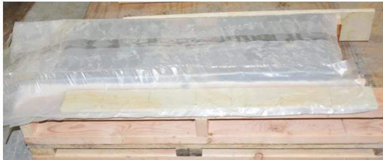
**Figure 7.10 Covering Freshly Placed Concrete Block with Plastic Sheets**
