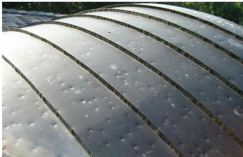
**Figure 4.2 Hail Dented Roof in Minneapolis (Kuhl 2019)**
