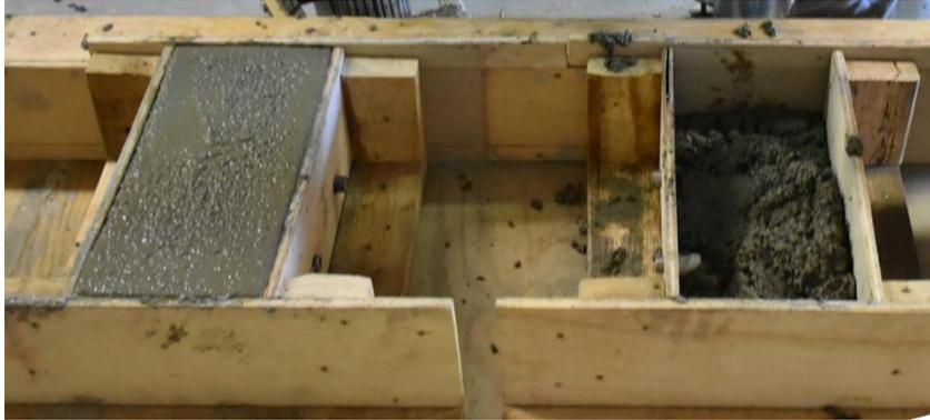
**Figure 7.9 Placing Concrete in the Formwork**
