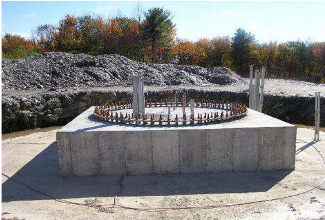
Figure 1.1: Wind Turbine concrete foundation with anchor bolts (Ceren, 2013)
